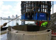
O-cell at the end of reinforcement cage
